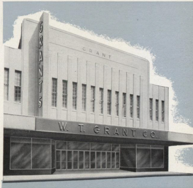
The Miami store at 9 E. Flagler Street has a second floor that extends to the corner. Another customer entrance opens to North Miami Avenue.
